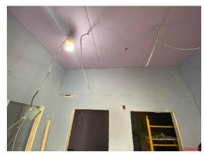
The weather has been brutally cold and windy, but progress continues on the restroom addition! The roofers completed installing the cedar roof, gutters, and soffits and started on the cedar siding. The interior of the addition is insulated. The carpenters have started hanging drywall and they are about 90% complete. Next week work will continue with plumbing, electric, and HVAC work.
